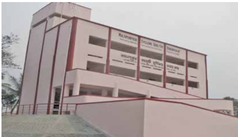
Construction of Cyclone Shelter at Haridashkati in North 24 Parganas District
