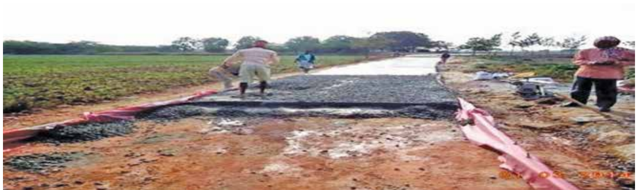
Connecting Cement Concrete Road in Ganjam District
