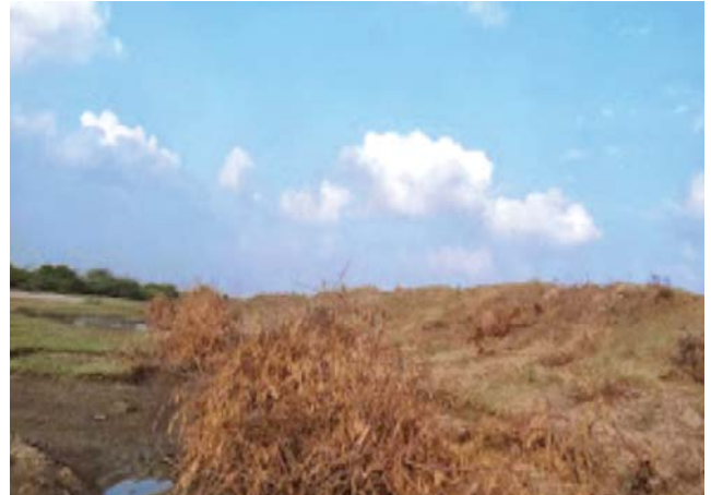
Kona Saline Embankment, Krishna District
