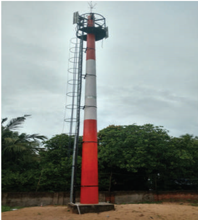
EWDS Spun tower, Ganjam, Odisha
