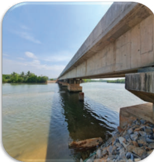
Evacuation route Bridge, Karnataka
