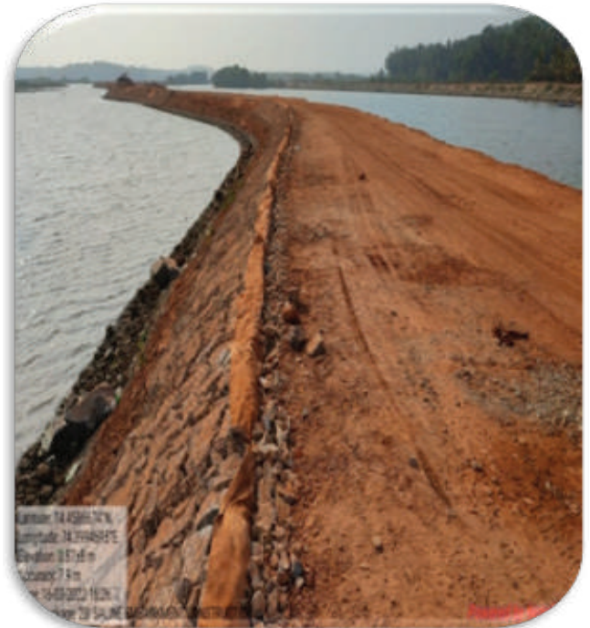
Saline Embankment, Karnataka
