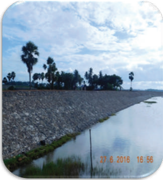
Saline Embankment, Odisha
