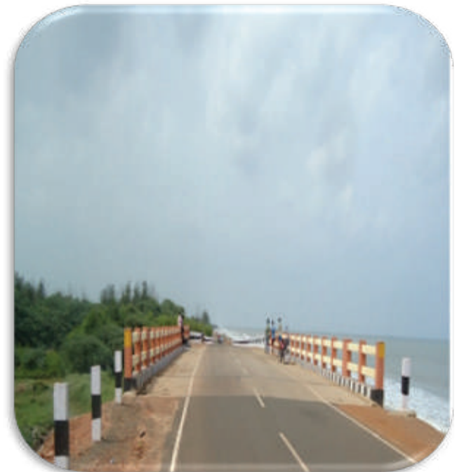
Evacuation route Bridge, Andhra Pradesh
